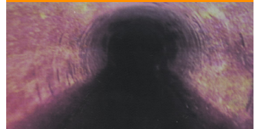
city pipe with grease
