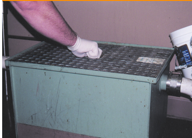
grease trap, hands on device
