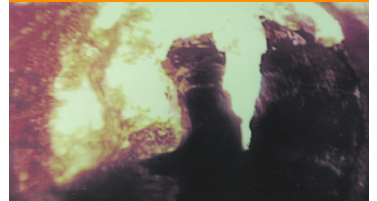
city pipe with grease
